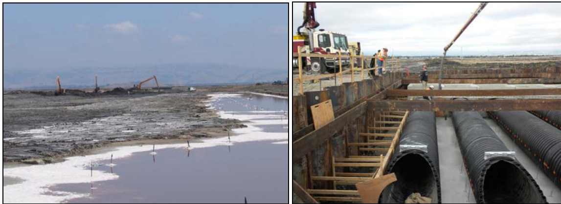
Pond SF2 Outlet Channel and Outlet Works Construction, August 2009
